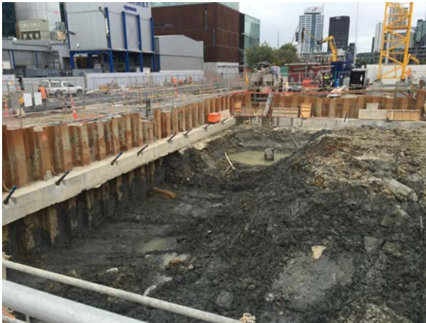
Figure 3: Concrete Waler Beam
