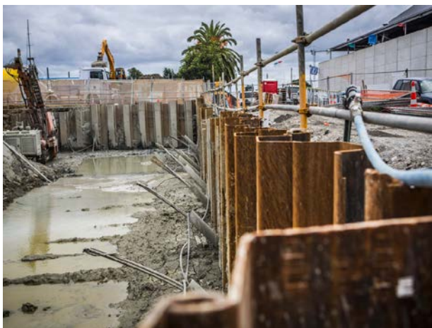
Figure 1: Sheet Pile and Anchor
