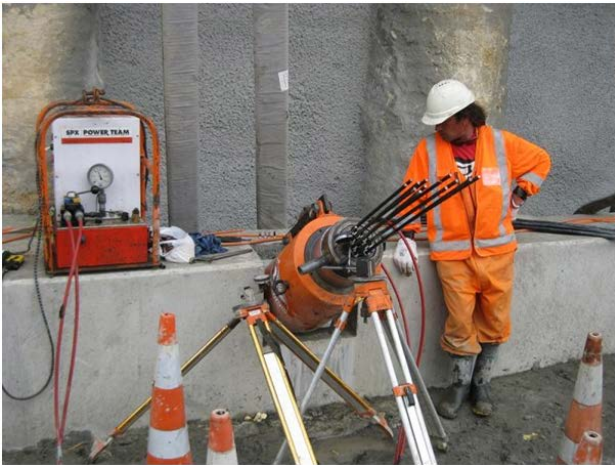
Figure 8: Typical Stressing Set Up
