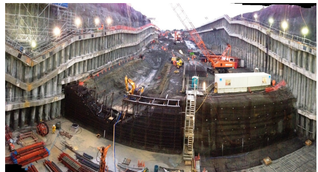
Figure 1: Southern Approach Trench
