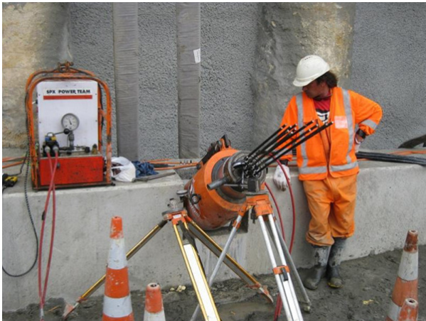
Figure 5: Stressing Set Up
