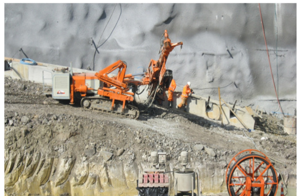
Figure 3: Specialist Anchor Drilling Equipment HD180 Anchoring Rig
