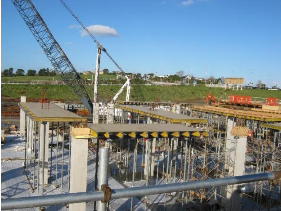
Figure 8: Doka Formwork System
