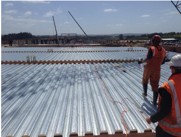
Figure 11: Comflor Permanent Soffit Formwork
