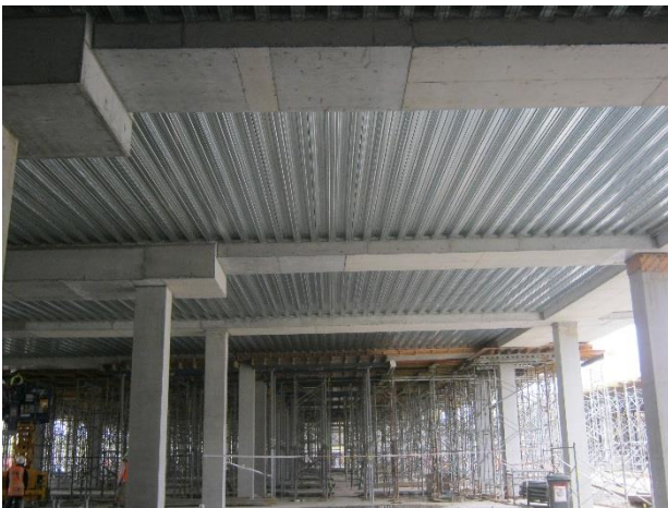
Figure 17: Stripped Floor Soffit
