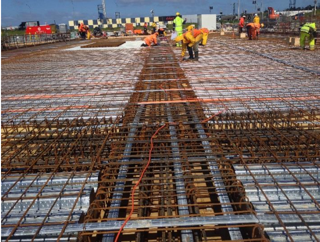
Figure 14: Post-tensioning & Reinforcement
