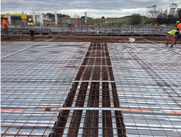
Figure 12: Post-tensioning & Reinforcement
