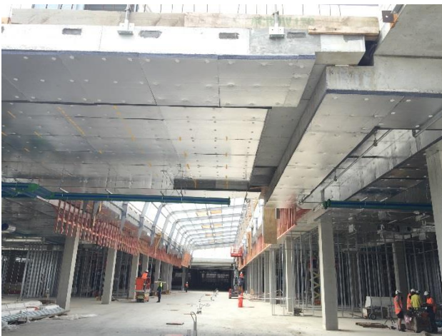
Figure 15: Corbel & Seismic Joint
