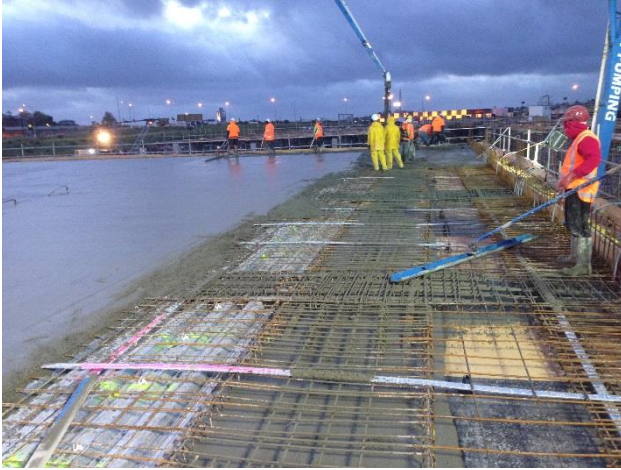
Figure 16: Concrete Pumping & Placing
