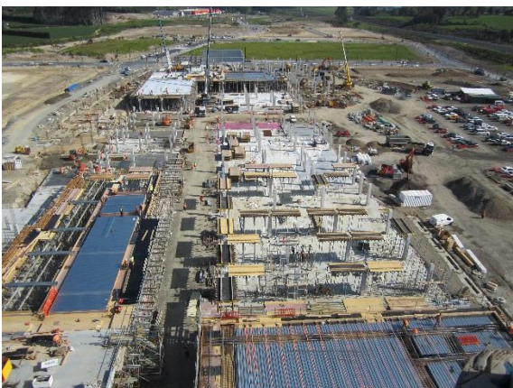
Figure 10: Multiple Work Faces
