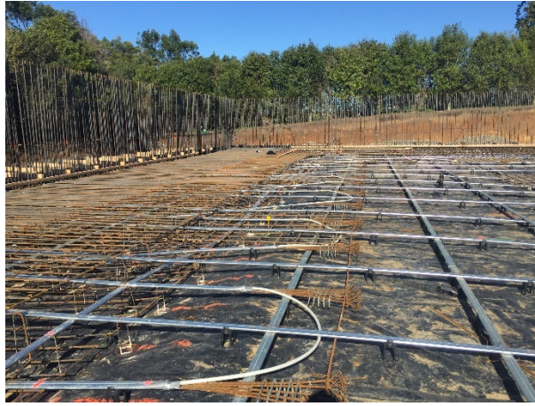
Figure 8: Post tensioning and conventional reinforcement
