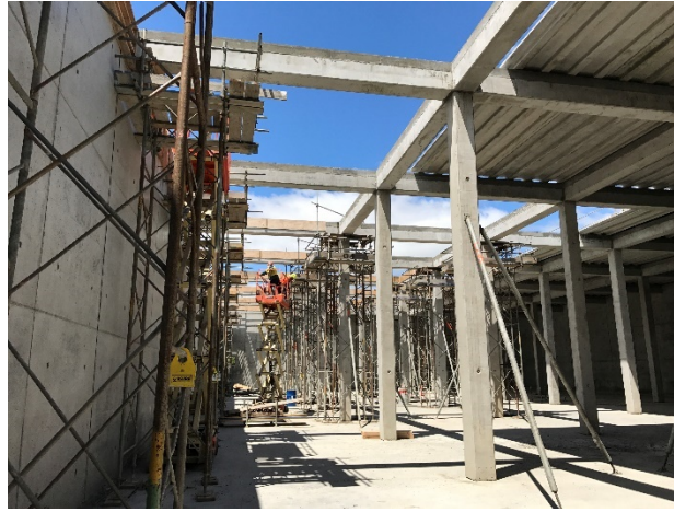
Figure 14. Precast columns, in-situ roof beams and unispan ribs
