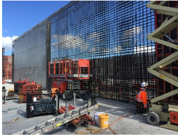
Figure 6: Wall prepared with post tensioning ducts
