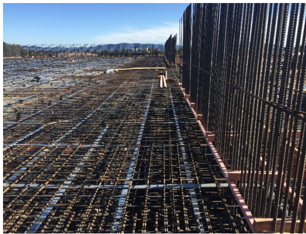
Figure 9: Reinforcement congestion
