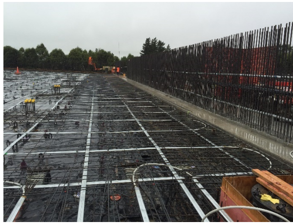
Figure 4. Coupled construction joint
