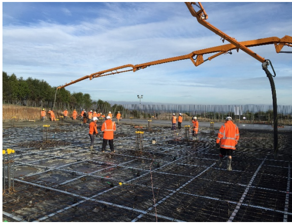
Figure 10: Concrete pumping and placement
