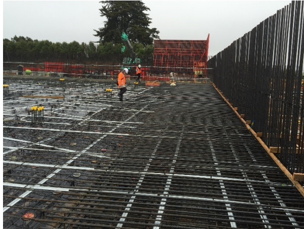
Figure 3. Perimeter thickening and reinforcement
