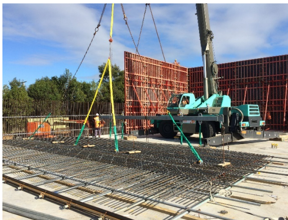
Figure 11: Wall reinforcement and Peri formwork
