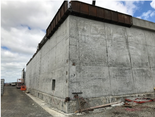
Figure 12. Completed wall off the form
