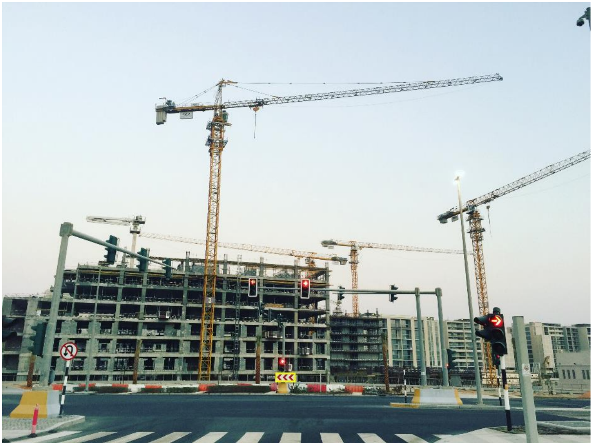
Typical Suspended Slab Construction - Middle East
