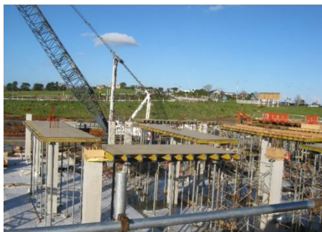
Elevated Height Falsework and Beam Soffit Formwork
