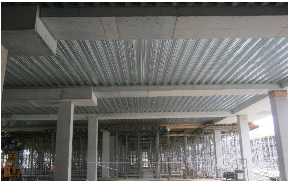
Typical Permanent Metal Deck
