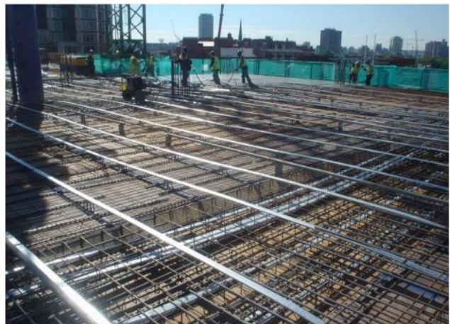
Typical Banded Slab
