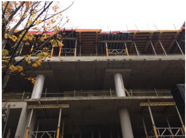
Typical Flat Slab with Drop Panels
