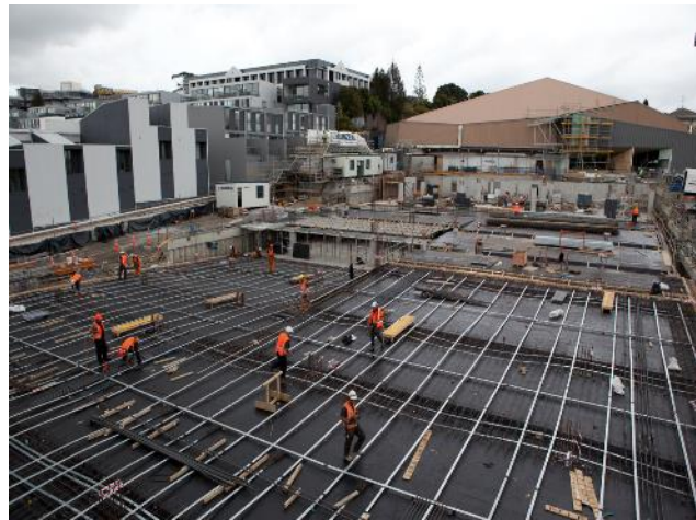
Typical Soffit Formwork
