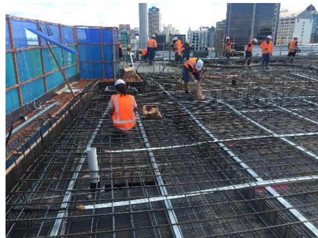
Typical Reinforcement in Suspended Slab - Apartment
