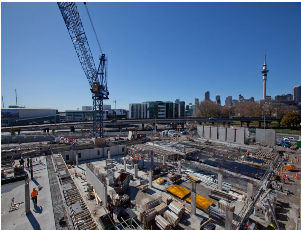
Typical Suspended Slab Construction - New Zealand
