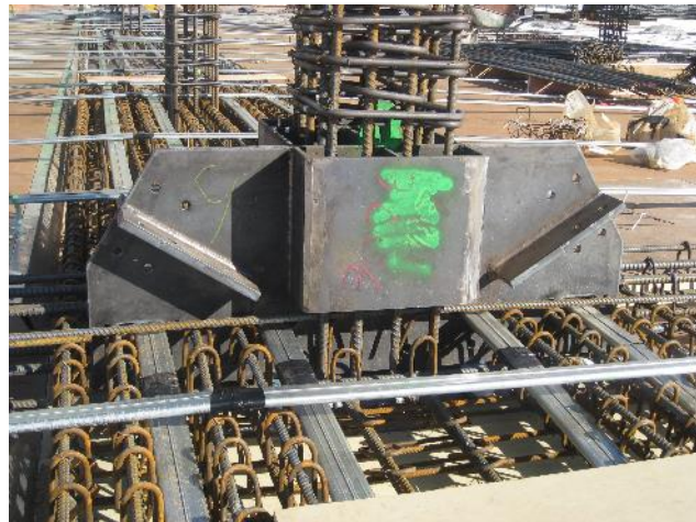
Congestion at Beam Column Joint with Seismic Brace
