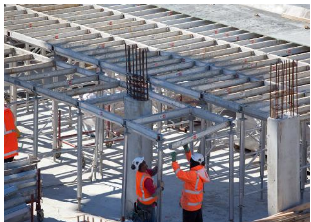
Aluminium Soffit Falsework
