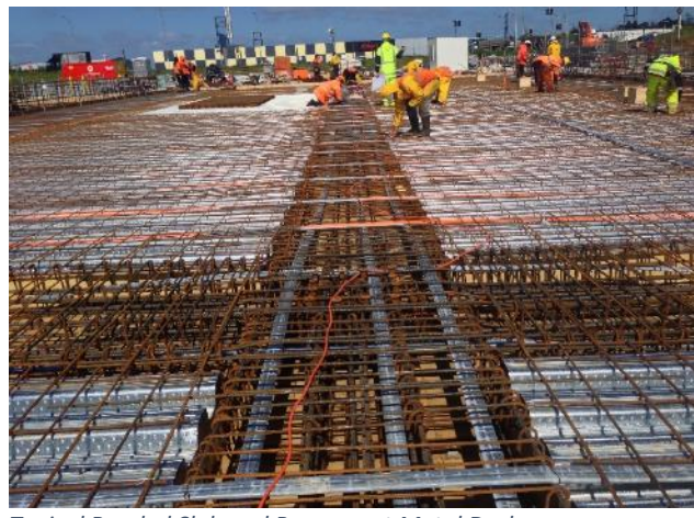
Typical Banded Slab and Permanent Metal Deck
