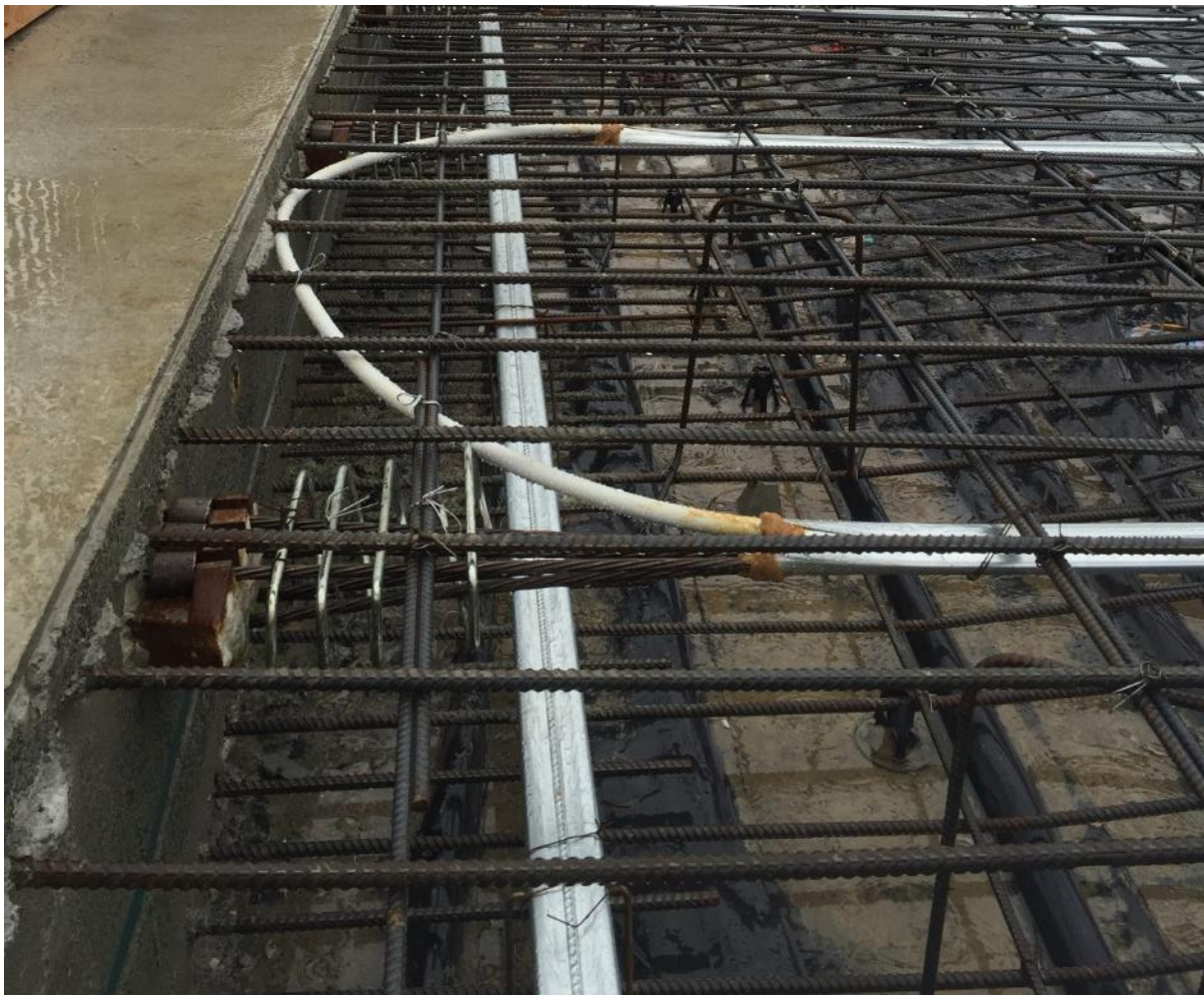
Typical PT Coupled Construction Joint
