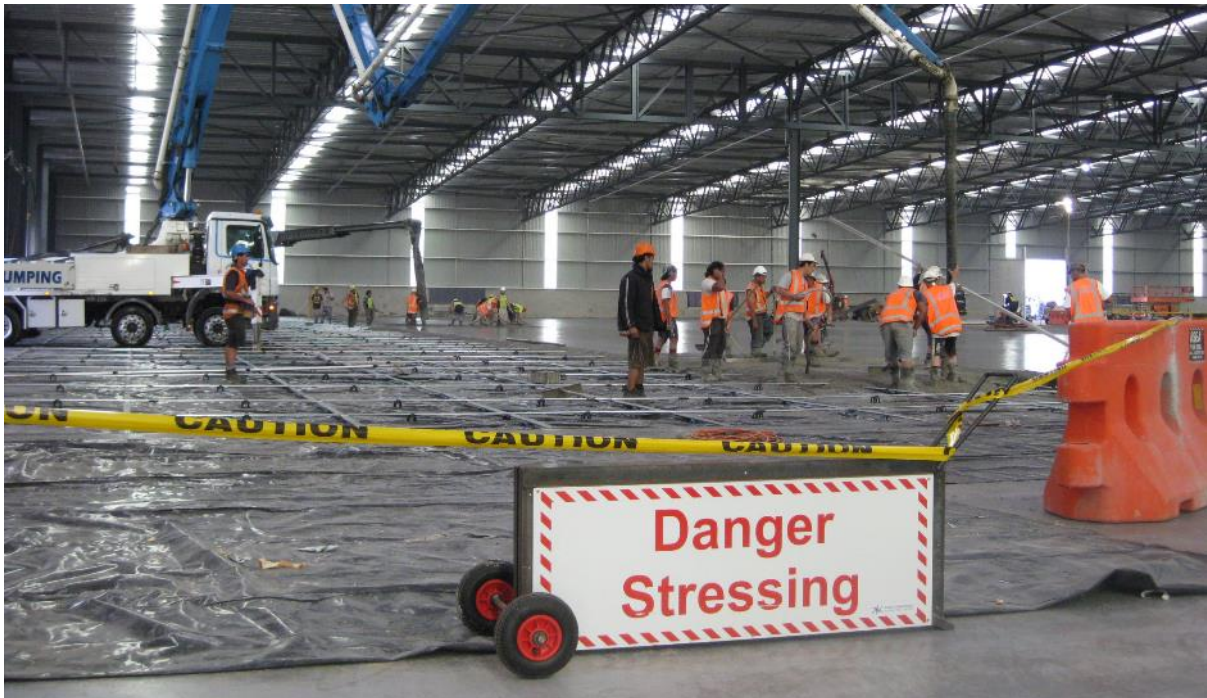
Typical Concrete Placing
