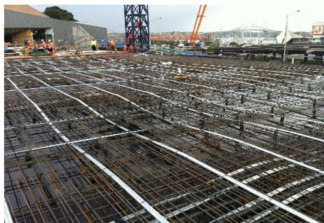
Typical Reinforcement in Suspended Slab - Carpark
