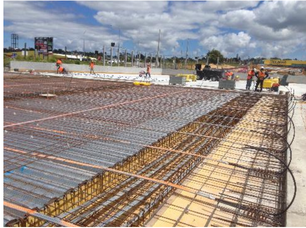
Typical Construction Joint Reinforcement
