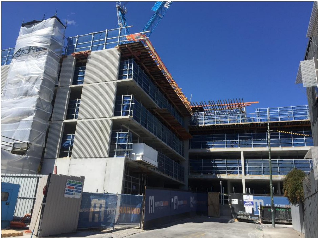
Typical Suspended Slab Construction - Australia
