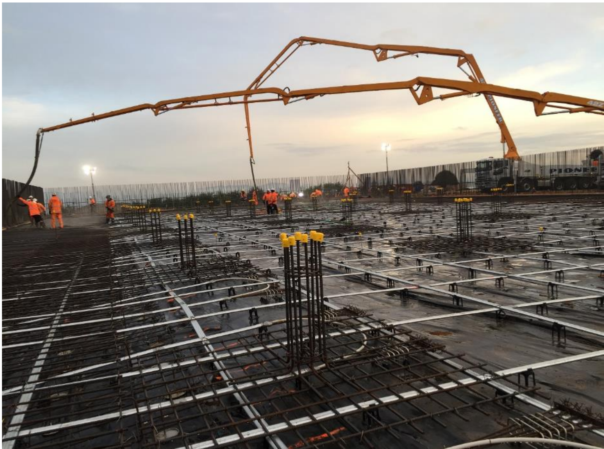
Rototuna Reservoir, Hamilton, New Zealand
