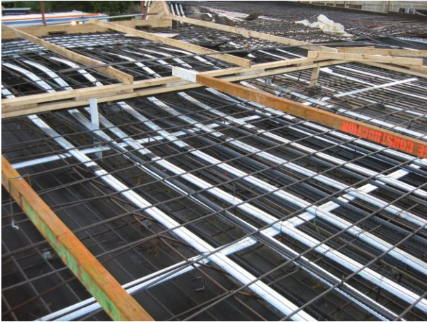
Figure 10: Post-tensioning and Reinforcement
