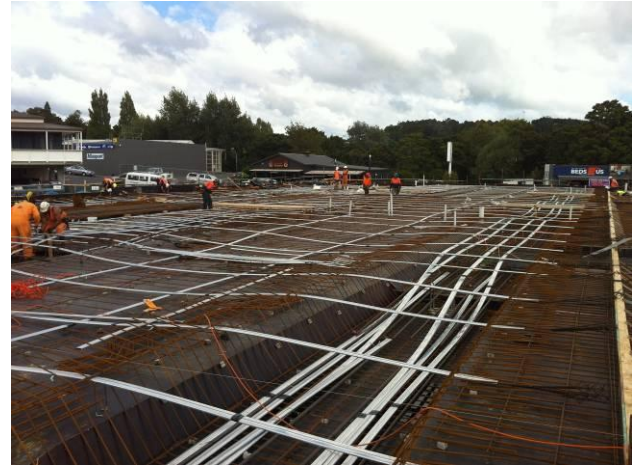
Figure 12: Post-tensioning & Reinforcement
