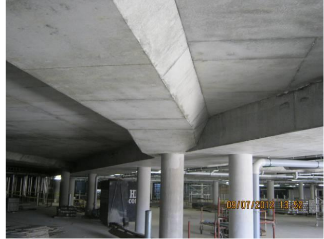
Figure 15: Recently stripped floor
