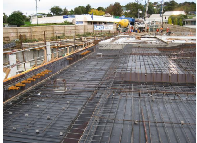
Figure 9: Complexity of Formwork
