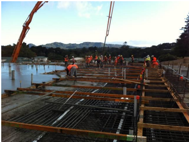
Figure 14: Concrete pumping and placing
