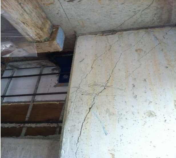
Figure 16: Restraint cracking within column
