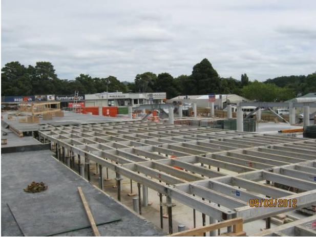
Figure 8: Ischebeck Formwork System
